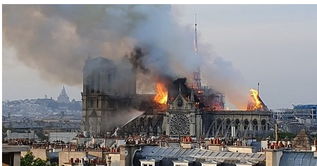
Figure 1. The Notre-Dame de Paris cathedral during the fire on April 15th 2019 (source : creative commons, author Marind)
