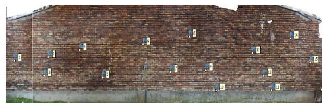
Figure 8. GCP locations (blue flags) on an unfolded image of the rounded tower (outside).
