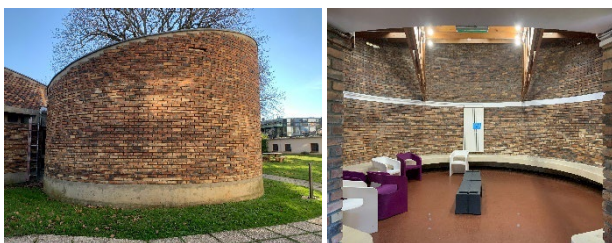
Figure 5. Tested cylindrical tower : outside and inside.
