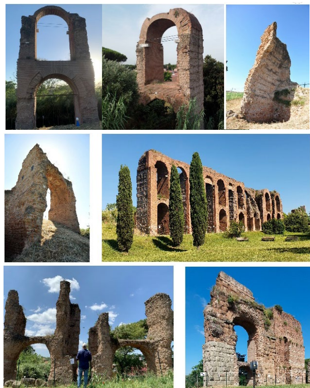
Figure 3 Sections A-G of Claudius-Anio Novus aqueduct in Tor Fiscale Park, Rome.
