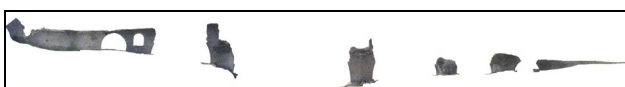
Figure 10. View 2 of the bridge current condition (remain of the bridge) (source: AutoCAD 2023)
