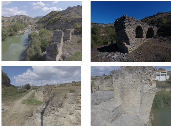
Figure 3. Bridge's current remains. (source: Photos from field survey)
