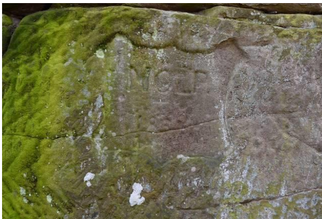
Figure 6. Almost illegible graffiti due to biological coating.
