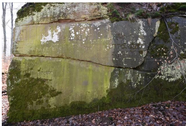
Figure 3. A stone wall of the quarry with graffiti and biological coating (moss, lichen, small tree) and water drainage traces especially on the right side.
