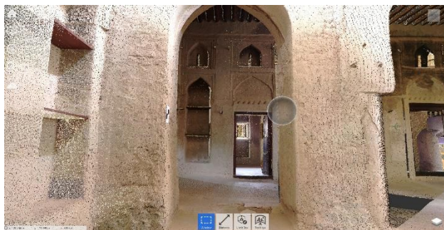
Figure 8. Point cloud of building interior taken with 3D scanner (2023).
