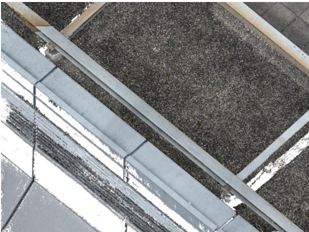
Figure 9. Detail of the upper part of the drone survey, showing varying results depending on the surface type and weathering
