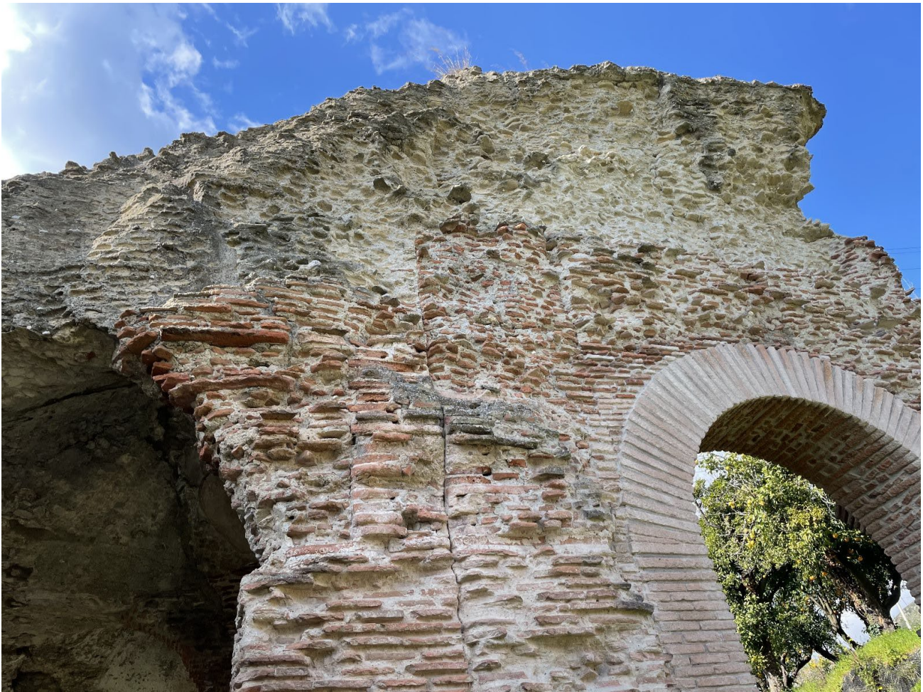
Figure 20. View of the outer wall of the ambulacro. Note that the two masonries are not joined
