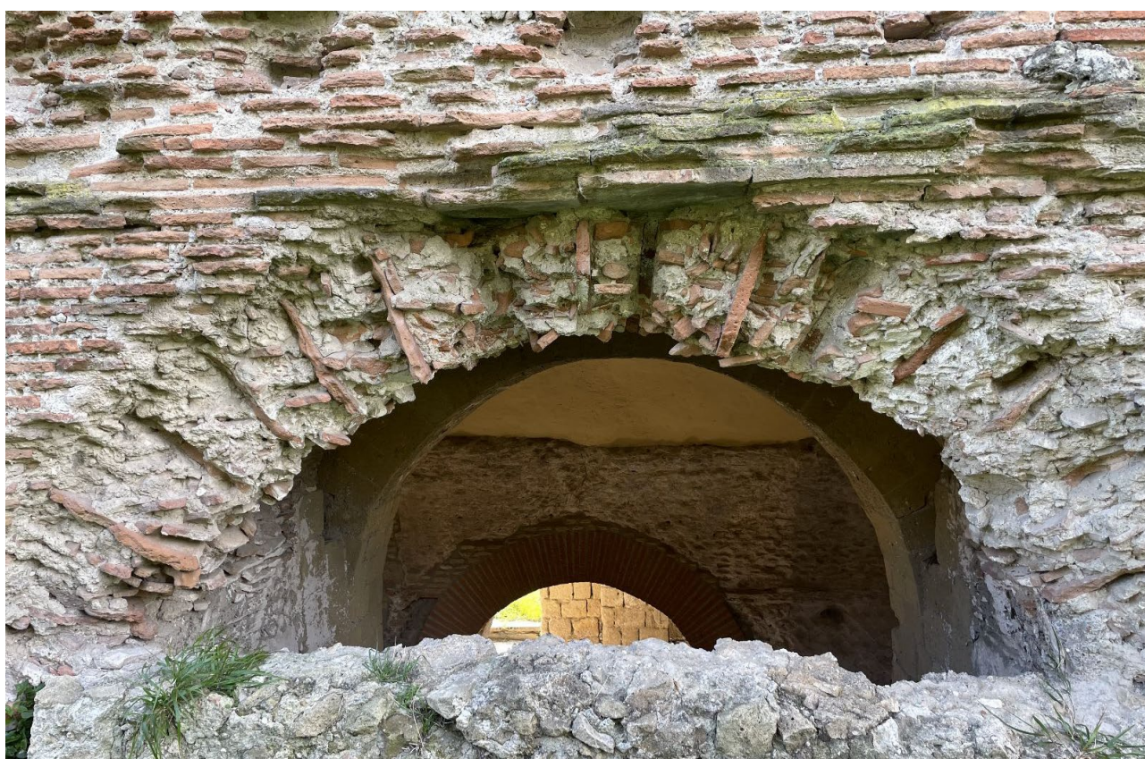
Figure 18. View of arches of the façade of the ambulatory
