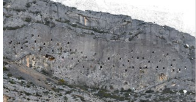
Figure 2. Covetes dels Moros. Bocairente. Dense cloud from terrestrial photogrammetry. Data processing in Metashape-Pro.
