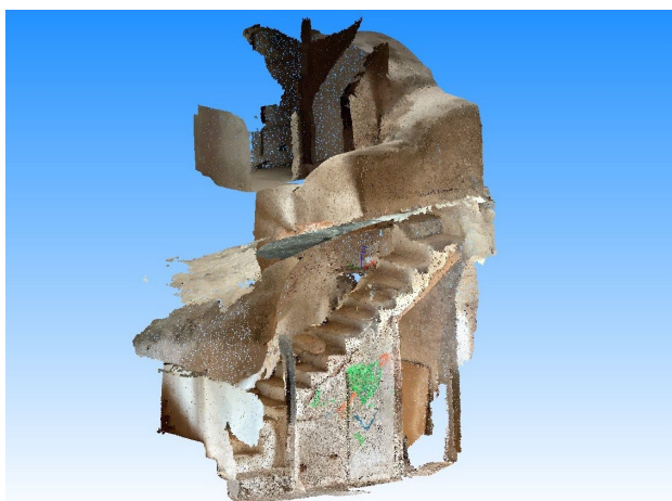
Figure 5. Cloud of 1.445.466 points of the staircase of the ground floor of the Rame tower, obtained with 3D scanner app installed on iPad Pro.
