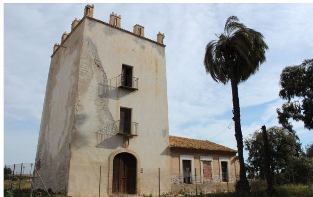
Figure 2. South facade and west facade of the Rame Tower. Current condition.
