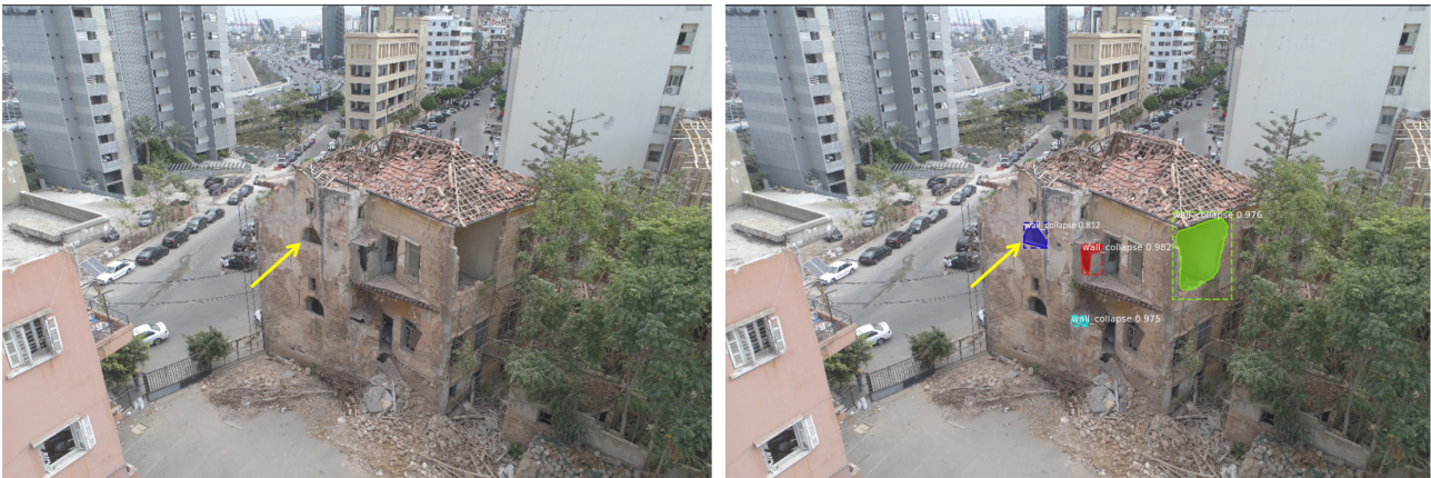
Figure 7. Photos showing the wrong detection of the wall collapse damage due to the similarity of demolished windows with actual wall collapse damage.
