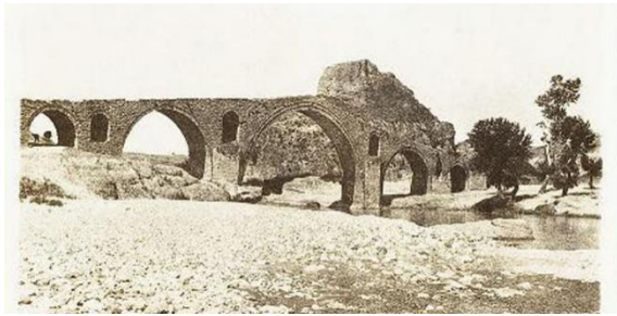
Figure 3. South view of the bridge before its collapse
