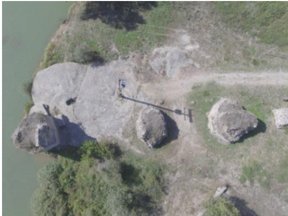
Figure 4. Top view of existing parts of the piers
