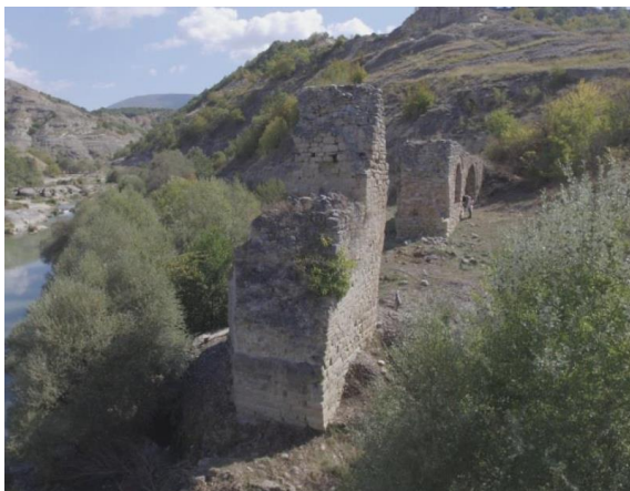
Figure 5. Side view of existing parts of the piers
