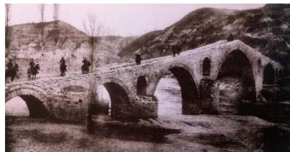
Figure 2. North view of the bridge before its collapse
