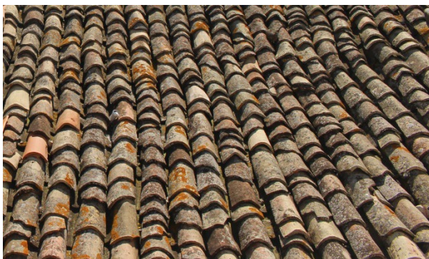
Figure 5. Ortho-image of the roof of testing building n.3 (TB3)
