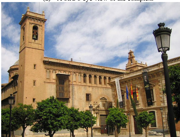
(c) The façade.
