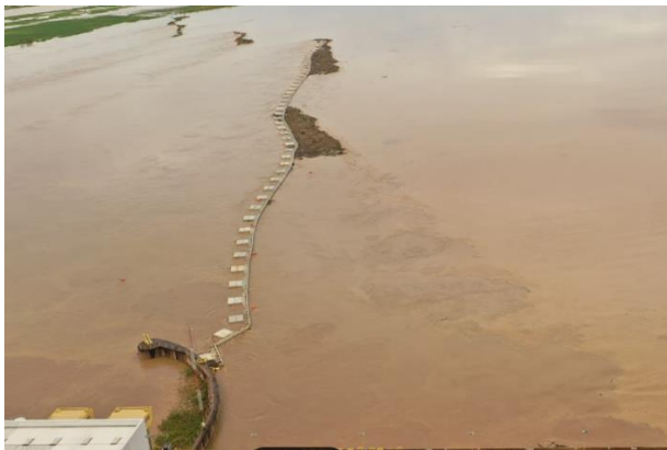
Figure 6 New log boom right bank
