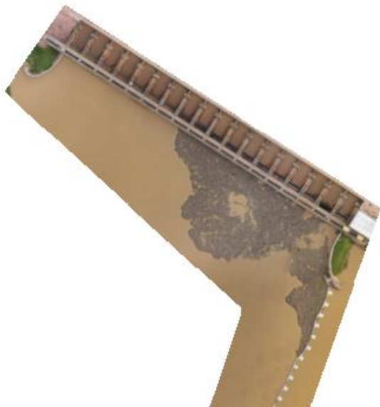
Figure 4. Orthophoto of spillway structure.
