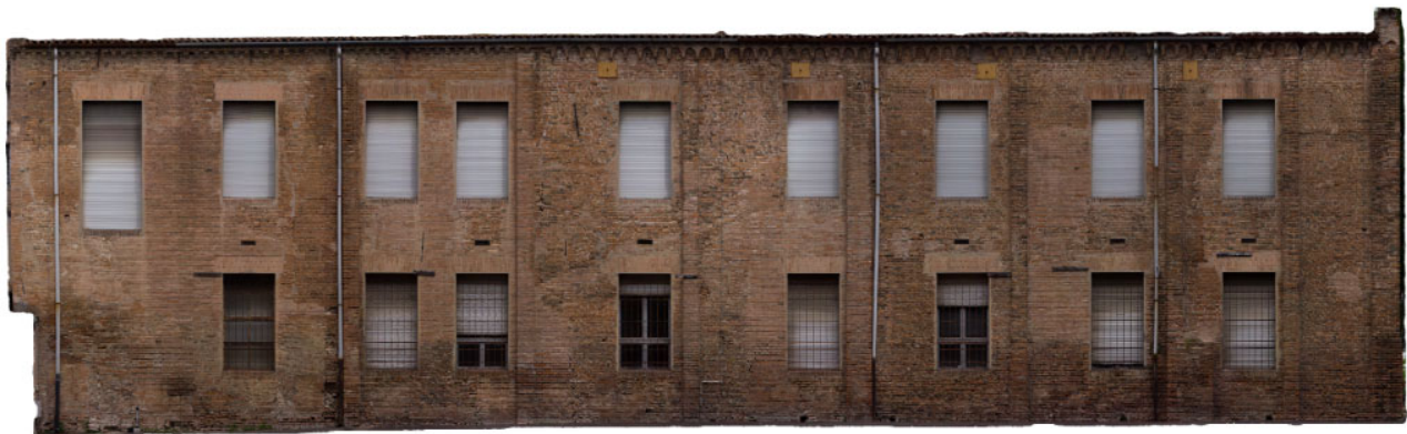
Figure 4. Former church of St. Catherine, south elevation. Orthomosaic processed in Agisoft Metashape®.
