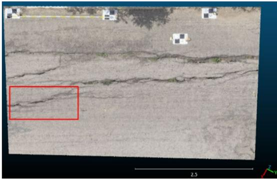
Figure 5. Longitudinal crack selected for the analysis.
