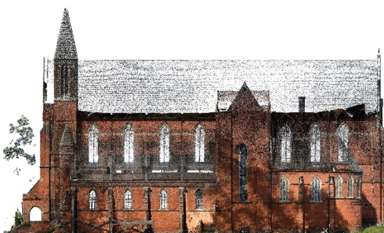
Figure 13: South elevation of St. John the Evangelist generated from point cloud data in RiPANO (RIEGL USA, 2020)
