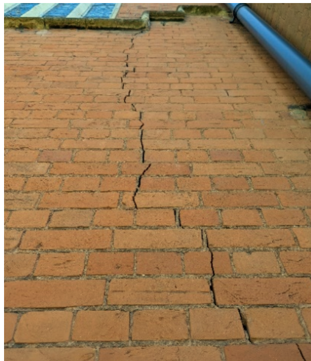
Figure 4. St John the Evangelist, Norwood Vertical crack in the south wall indicating possible settlement
