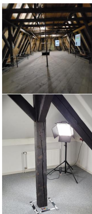
Figure 4: Heritage roof framework in Bamberg (top) and the wooden beam at the Jade University of Applied Sciences showing diffuse lighting of dataset D (bottom).
