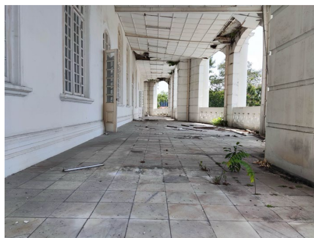
Figure 17. Sloping floor of verandah in Ipoh Town Hall and Post Office on site.
