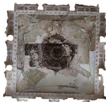
Figure 5. The orthomosaic of the damaged atrium produced using the photogrammetric method. (©UNESCO/ICOMOS)
