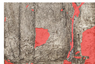
Figure 8. Identified bridge damage.
