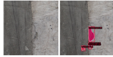
Figure 4. Examples of damage recognized by Mask R-CNN.
