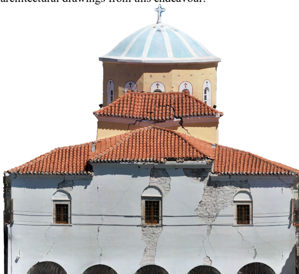
Figure 9. East View facade ortho-image depicting damages in Dormition of the Virgin Mary in Ano Bathy
