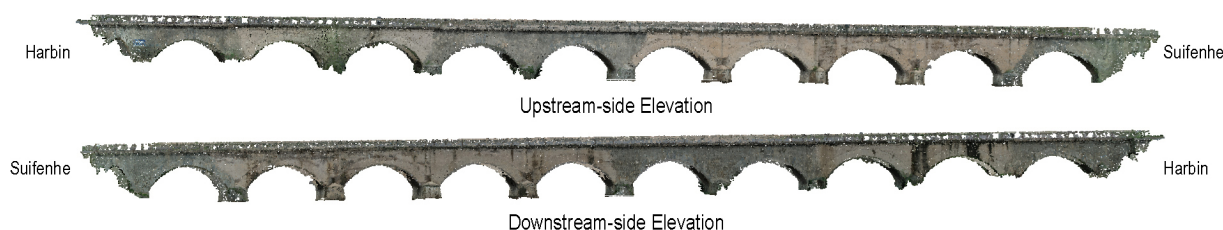
Figure 5. Raw point cloud data illustrating the elevation profiles in both directions of the bridge.
