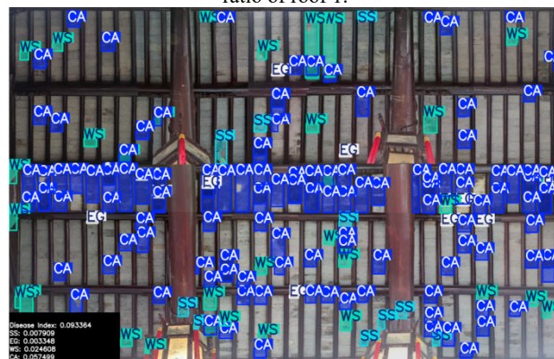
Figure 12. Quantitative detection results and pathology area ratio of roof 1.
