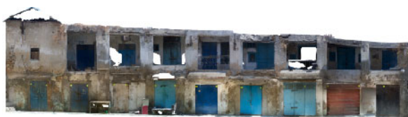
Figure 3. Photogrammetric model of the façade, showing control points (yellow signs) at the corners of door openings. Gaps indicate areas that could not be captured due to visibility.
