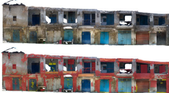
Figure 6. Conservation state of building elements. The top image shows the original condition, while the bottom shows damage mapping by priority. Damage levels are indicated by colour, as defined in Figure 7.
