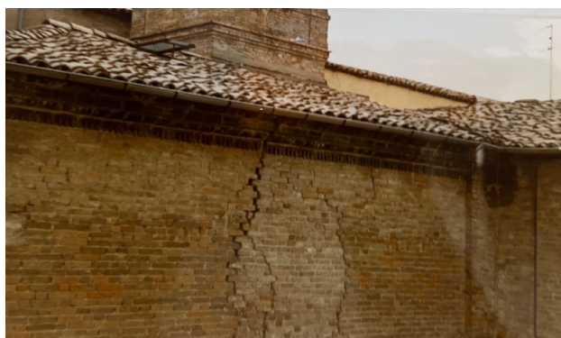
Figure 8. Seismic damages occurred on the façade (top image) and the not-confined nave wall (bottom image) during the 1983 earthquake (Privitera, 2025; SABAP-PR, PR/M 37)
