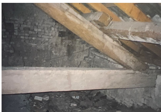
Figure 9. Seismic damages occurred on the façade during the 1996 earthquake (Privitera, 2025; SABAP-PR, PR/M 37)
