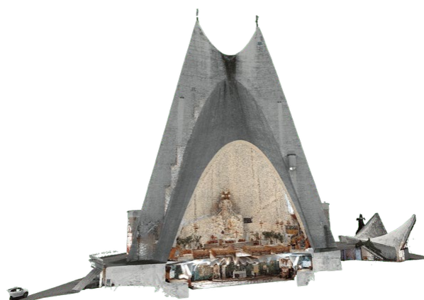
Figure 5. Divine Mercy Church in Kalisz (cross-section through a point cloud) (K.Argasinski/BIMfaktoria, 2025).
