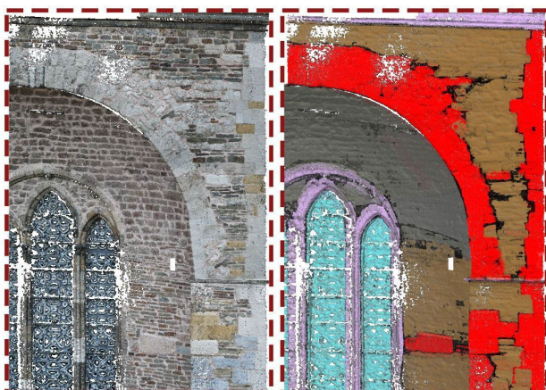
Figure 10. Portion of the reprojection on the photogrammetric model of the semantic masks generated via SAM (elaboration by the authors).
