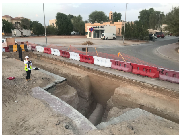
Figure 2. Excavation of a falaj shaft emerging beneath modern urban infrastructure.
