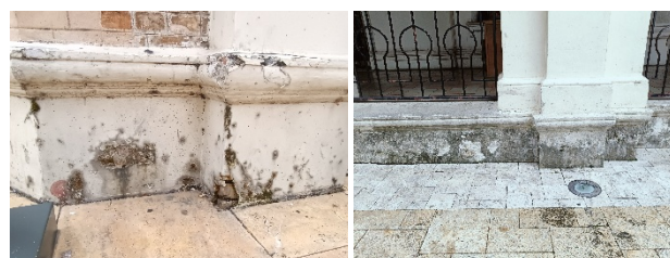
Figure 16. Water damage in the Wall and Foundation
