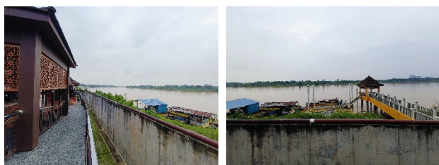
Figure 5. Flood barrier along the Kelantan River protecting the Masjid Kampung Laut. (Source: Author)
