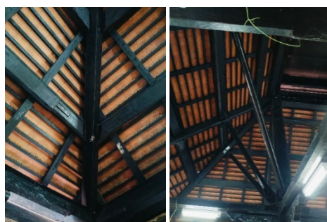
Figure 10. The mortise-and-tenon join for roof trusses is now supported with a metal structure to strengthen the roof. (Source: Author)
