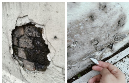
Figure 17. The wall cracked, and plaster spalled.
