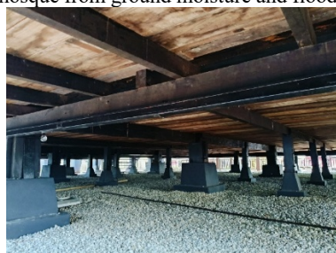
Figure 6. The original 20 structure pillars were supported with modern concrete footing. (Source: Author)
