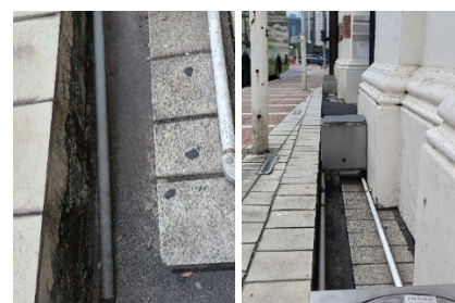
Figure 15. Additional components (Spotlight and piping) were obstructing the existing drainage
