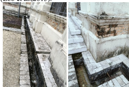
Figure 14. Poor perimeter drainage system of Bangunan Sultan Abdul Samad (Source: Author)
