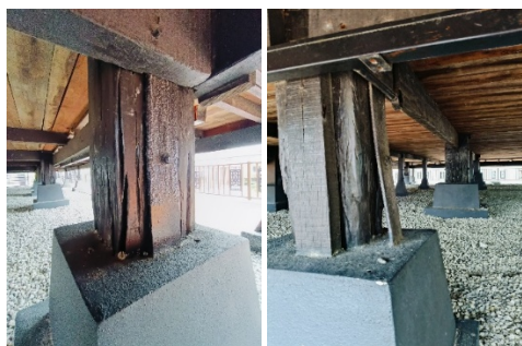
Figure 7. The timber pillar foundation was supported with a metal support. (Source: Author)
