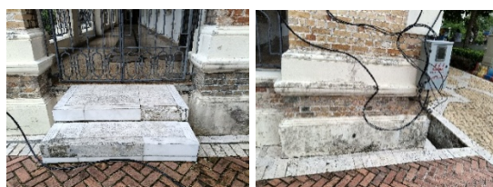
Figure 18. Additional electrical DB and conduit exposed to public access. (Source: Author)
