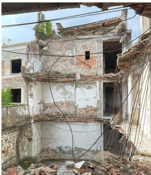
Figure 3. View of a portion of Colonia Varese affected by collapses of horizontal structures (photo by the authors).
