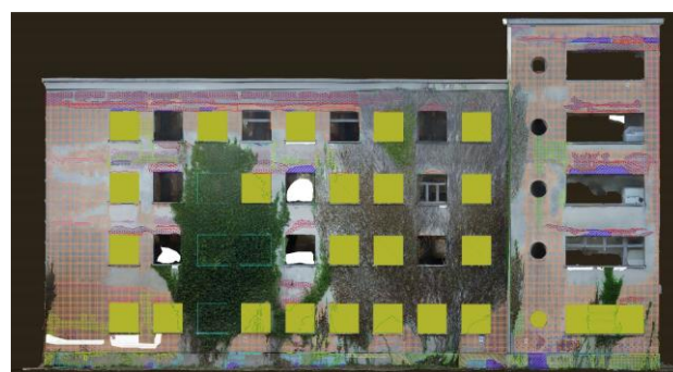
Figure 13. Sample of degradation outlining on the surfaces of one of the elevations, using the DEM as a basis for mapping the conservation conditions in detail (graphic elaboration by the authors).
