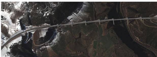
Figure 9: Pleiades-HR sensor image of Viaduc de Millau, © CNES Copyright 2012
