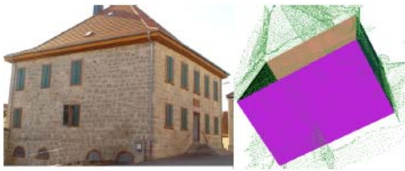
Figure 8: Left: Image of building consisting of four major walls standing on a slope. Right: The derived point cloud consists of 273 000 points, the four major walls were successfully detected, segmented and connected.
