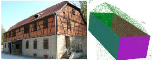
Figure 9: Left: Image of building consisting of four major walls having a dominant entrance and stairs at one side. Right: The derived point cloud consists of 271 000 points, the four major walls were successfully detected, segmented and connected.
