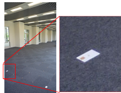
Figure 8. RFID tags installed on the floor
