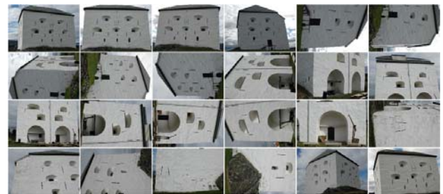
Figure 14. Overview of 24 photographs used for automatic texture mapping of the 3D building model of fortress Kristiansten in Trondheim
