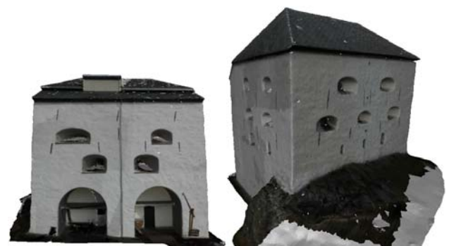
Figure 15. Perspective views of the automatically textured 3D building model of fortress Kristiansten
