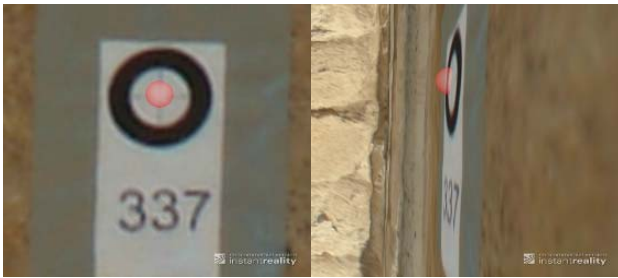
Figure 8. Superimposition of control points in the textured 3D model for geometrical quality control
