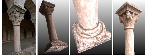
Figure 1: Image-based 3D reconstruction of a column with its decorated capital and basement.
