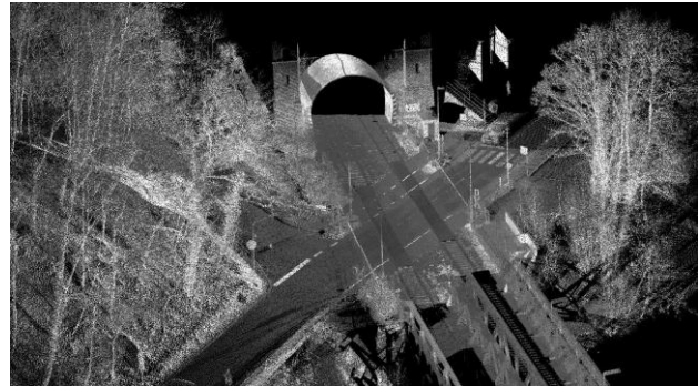
Figure 17: Point cloud of a railroad crossing
