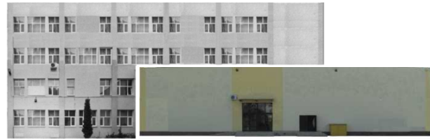
Figure 9. Rectified mosaic image of the north-east facade (from UMK raw images)
