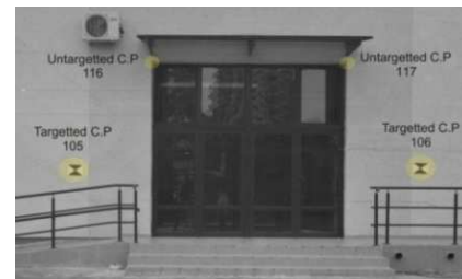
Figure 2. The location of some natural and artificial control points (North facade)
