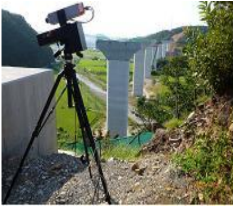
Figure 11. Photography using VNIR camera on Daejongchun Bridge
