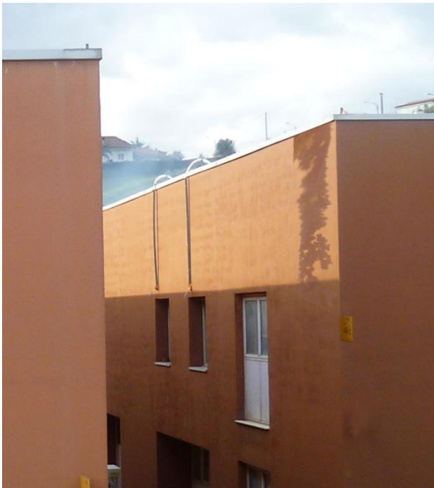
Figure 11. The new image of test 3
