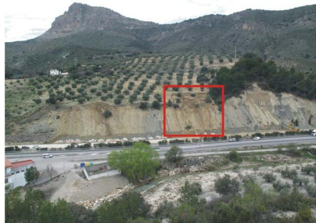
Figure 2. Panoramic photograph of studied landslide affecting road cut and upslope. The main scarp is inside the red square.
