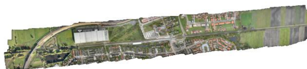
Figure 7 Orthomosaic of a metro station
