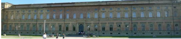
Figure 9. Northern façade of the Old Pinakothek
