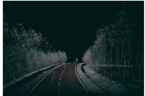
Figure 7. Scan result of a land road (206 meter)
