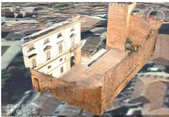
Figure 5 A Terrestrial Laser Scanner Point Cloud
