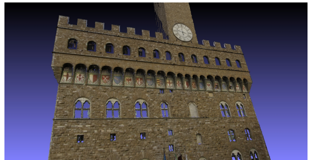
Figure 7. Color projection on the triangulated surface of the front of Palazzo Vecchio.
