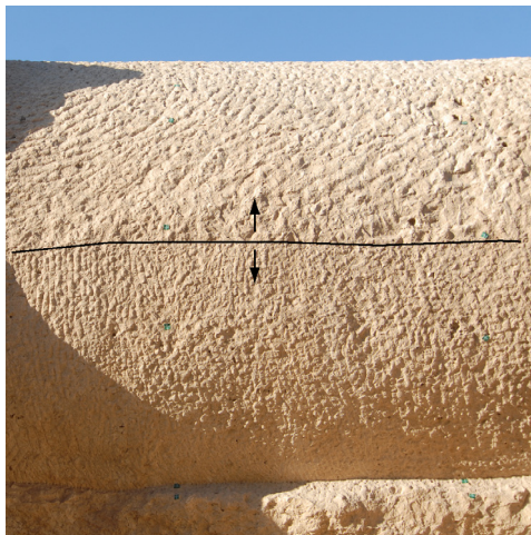
Figure 9. The border line of chisel marks on the south side
