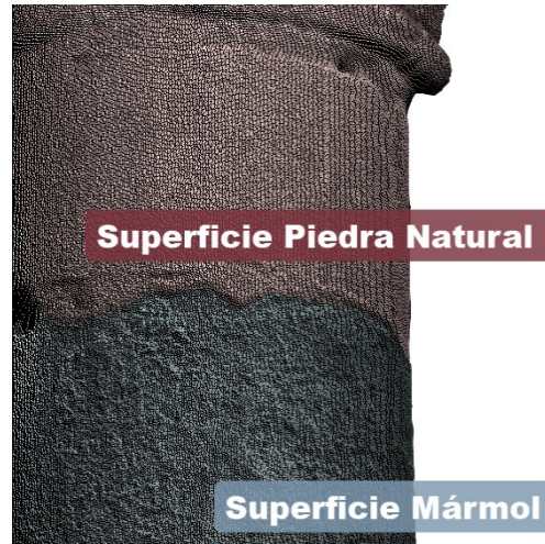
Figure 15. Despite of the model appearance, the finish of the entire shaft is the same for both stones.
