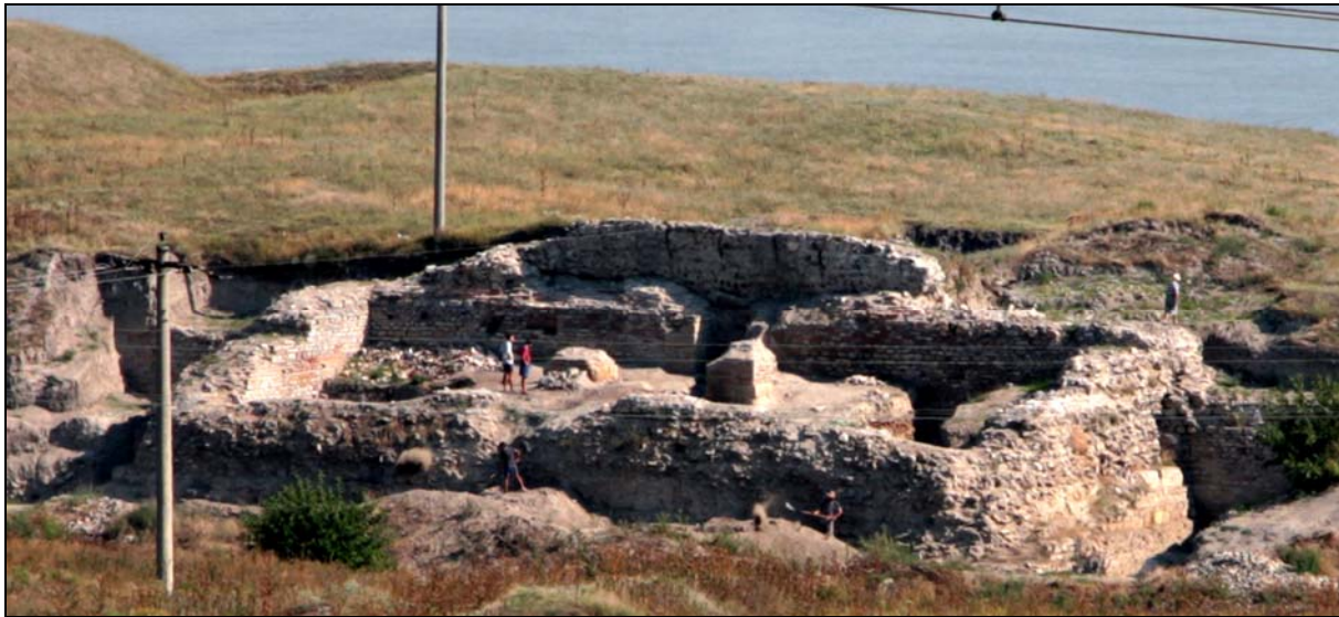
Figure 5. The Large Tower from Noviodunum measures 30.9 x 14.5 meters in plan; elevations are preserved to ca. 5 meters on the outside of the tower. The human scale as shown in this photograph may be more relevant.
